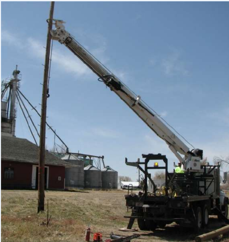
New telephone pole last April.
