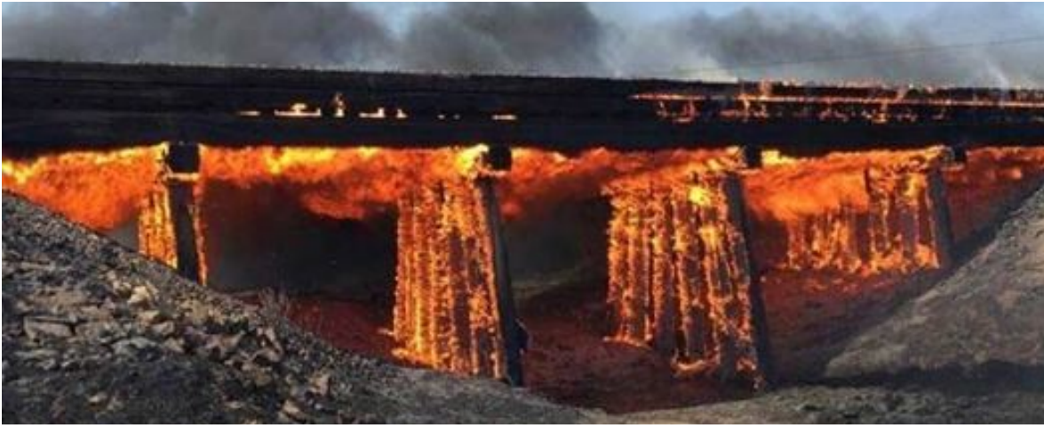
Arson caused old MOP / D&RGW trestle fire 2016. Otero Sheriff's Office picture.
