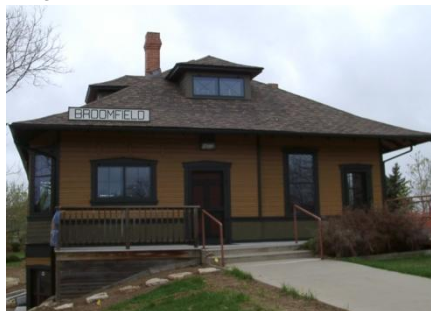
Above: The station agent's bay is visible at left, the main depot entrance is in the center, and the agent's quarters entrance is a separate door at the far right.
