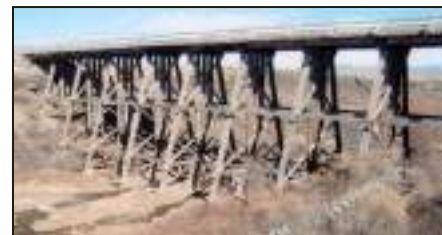
San Luis Valley Southern Railway Trestle, 2002
