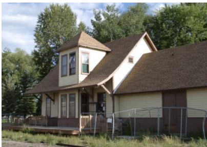
Monte Vista depot with platform from track side
