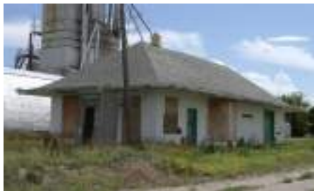
Angle view of the front and east side of depot
