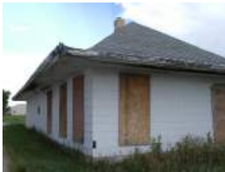
Angle view of back and east side of depot
