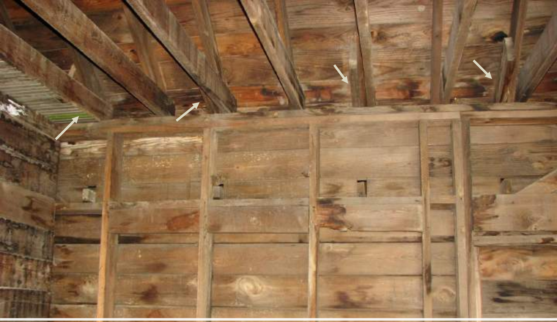
Soffit Rafters Within the Depot
