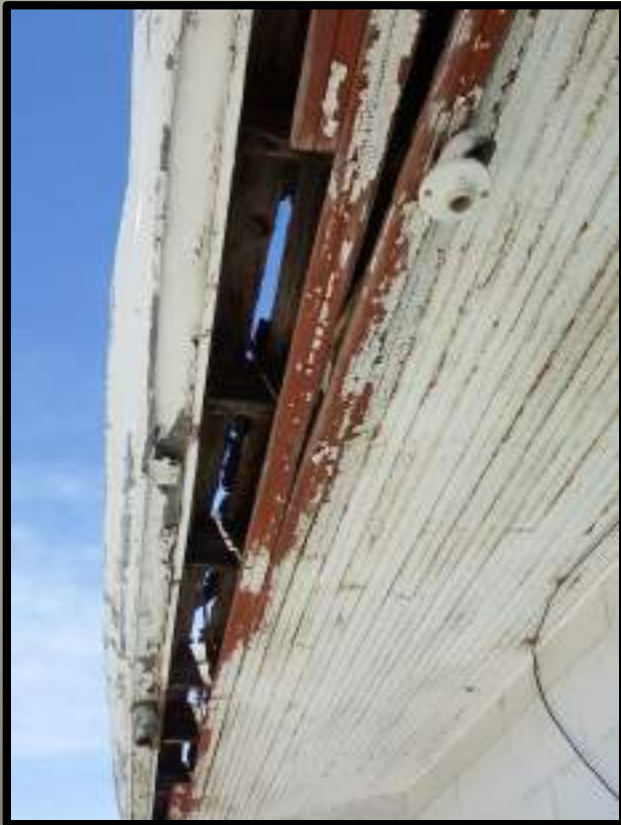
Roof, Gutter, & Soffit Concerns at the Depot
